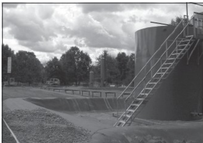
THE PRODUCTION FACILITY constructed for West Bay Exploration's Foote 1-12 well in Calhoun County's Marengo Township (T2S-R5W) is shown in the photo at left, taken in late September 2006. Reports from the field indicate that the well's success and its potential significance have spurred a flurry of leasing and exploration activity in the area.
